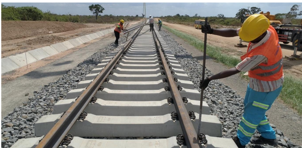
Figure 7: Laying of Phase I from Dar es salaam to Morogoro (205km) Standard Gauge Railway (SGR) (Courtesy: Government of the United Republic of Tanzania)
